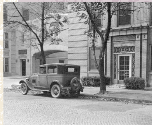
Original research building entrance
